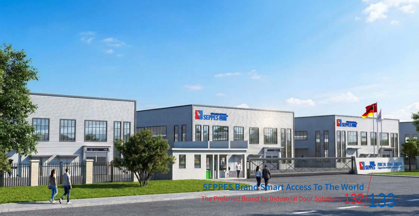
▼ The new factory in Seppes Door Industry, with a planned area of over 50,000 square meters
