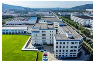
Aerial view of the SEPPES factory
