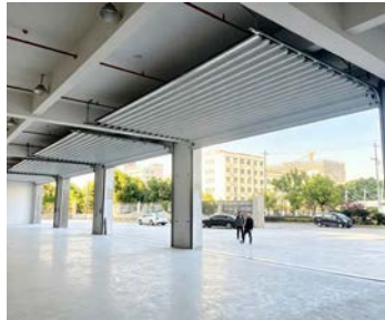
Rib-reinforced wind-resistance Sectional door
