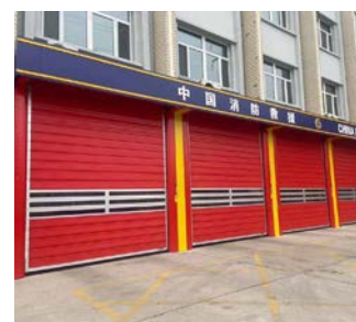
Fire station garage door
