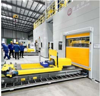
Production Line Interlock Control
