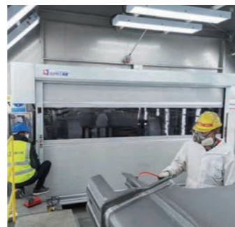
Painting equipment room
