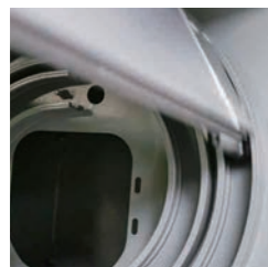
Turbine spiral suction structure
