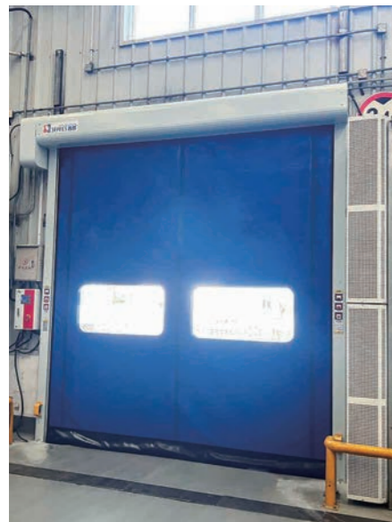
Dual air curtain linkage zipper quick door
