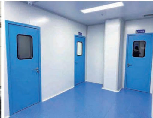
Steel swing door of the purification workshop
