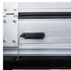
Wireless safety anti-pinch bottom edge
