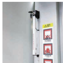
Power-off Manual release device
